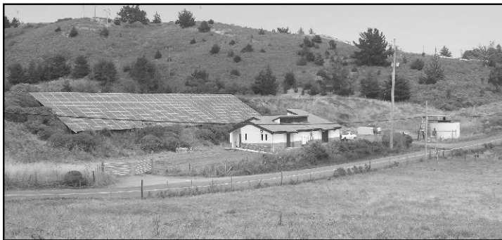
Woodrat Water Treatment Plant on Mesa Road
