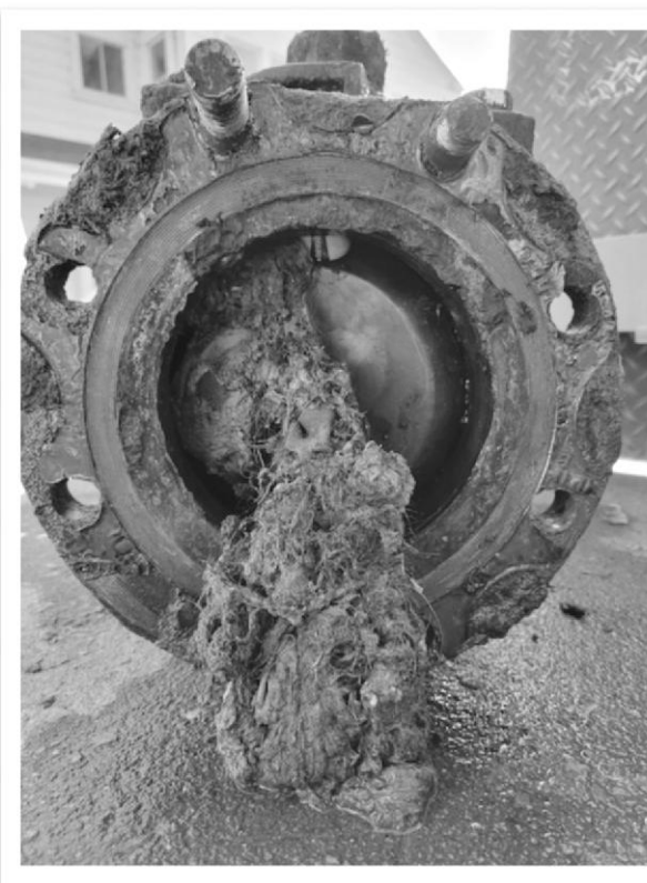
Wipes and rags obstructing a BCPUD check valve.
