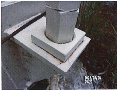
Anchor after sanding prior to prime coating.
