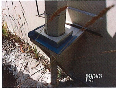
Anchor chairs with prime coat applied.
