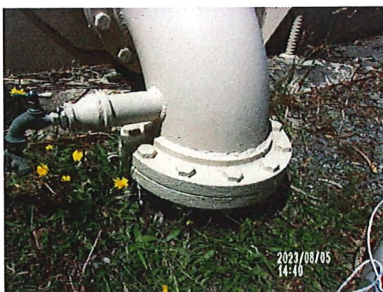
Bottom bolted flange after priming and finish coating.
