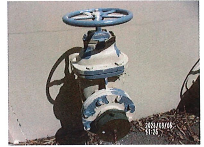
Valves with prime coat applied.
