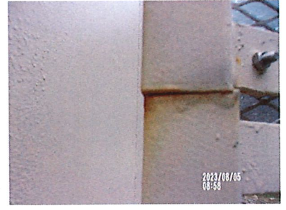
Ladder cage joint prior to sanding and caulking.
