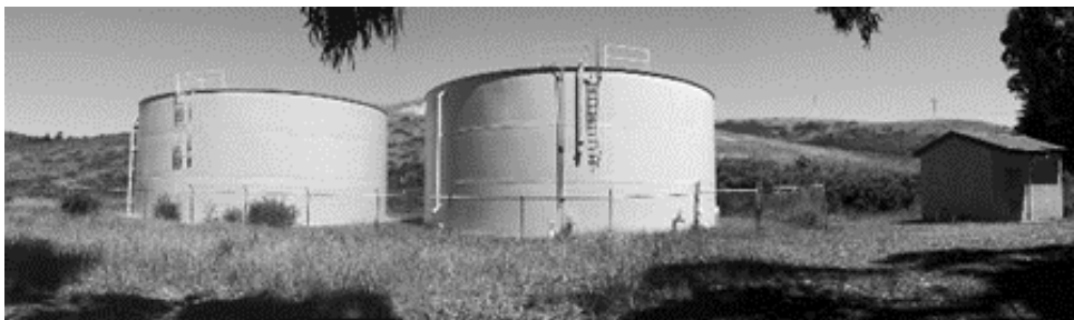
BCPUD's East and West Water Storage Tanks
