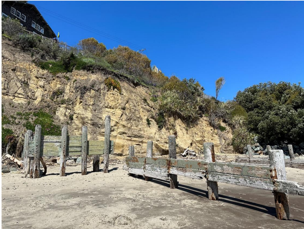
Photo 7: Remnants of timber groins to the east of the sea wall. Photo: IMG_0376.jpg Date: 4/13/23
