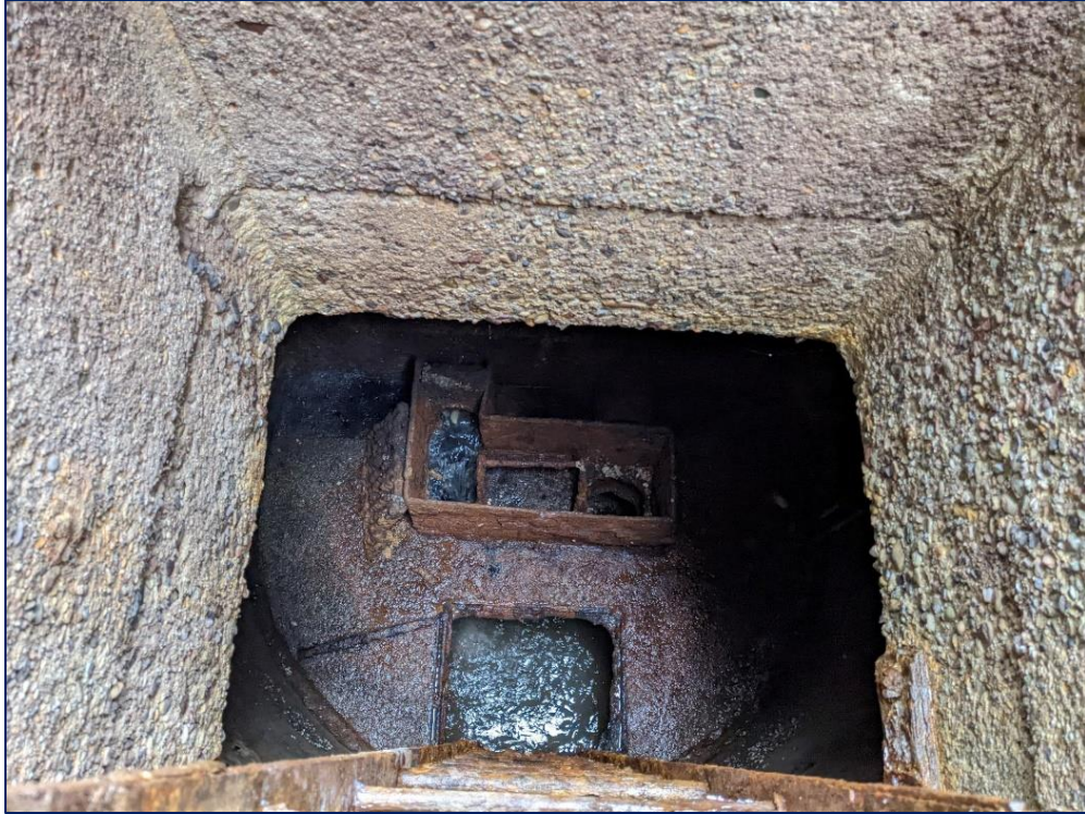
Existing Concrete Wet Well
