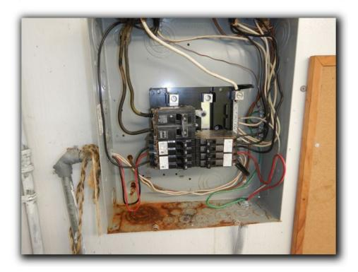
Not all of the circuits (breakers) in the panel were identified or labeled. We recommend all circuits be © 2024, BUTLER COMMERCIAL BUILDING INSPECTION INC.
