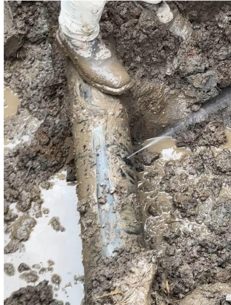
Leak on Booster Line
