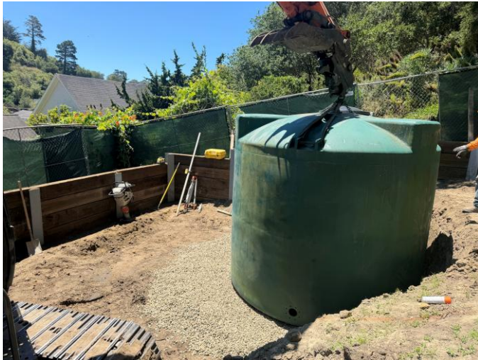
Well Project at 31 Wharf
